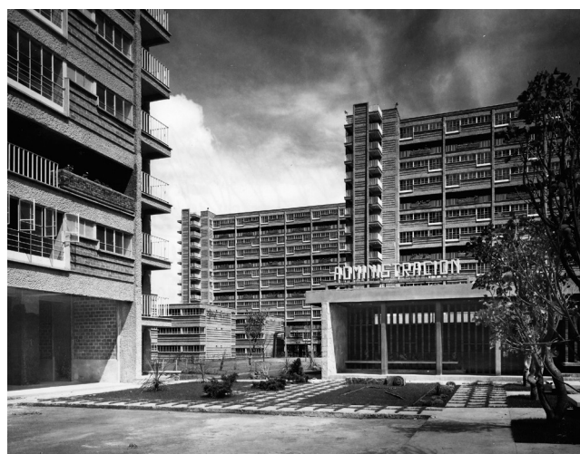
01 Mario Pani, Centro Urbano Presidente Alemán , Mexico City, Mexico, 1947-1949. Entrance to the administrative offices. © Guillermo Zamora, Archive Louise Noelle.
