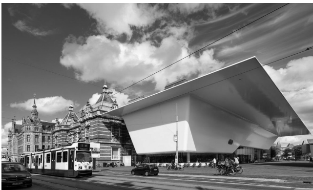
03 Benthem Crouwel Architekten, Stedelijk Museum extension, Amsterdam, The Netherlands, 2014. It features an innovative synthetic skin that is almost seamless. © Janne Linders.
